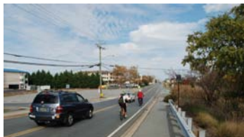
Figure 69 Difficult bicycling conditions along Savannah Road
