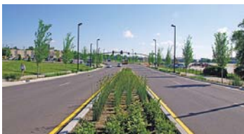
Figure 82 Example of narrow median with infiltration in Nashville, TN
