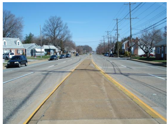
FIGURE 6: PAVED MEDIAN AND ON-STREET PARKING IN SHOULDER
