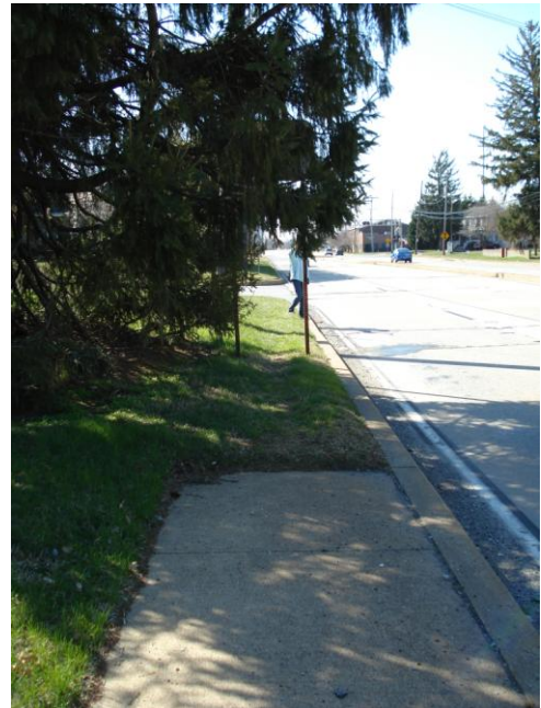
FIGURE 5: END OF SIDEWALK ON ROUTE 9 NORTHBOUND
