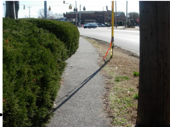
FIGURE 13: ENCROACHMENT OF NARROW PATH ALONG ROUTE 273 BY OVERGROWN SHRUBS
