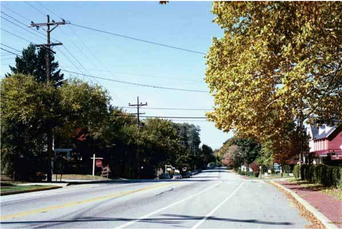
Figure 8 - Kennett Pike in the Village of Centreville, Segment 10.
