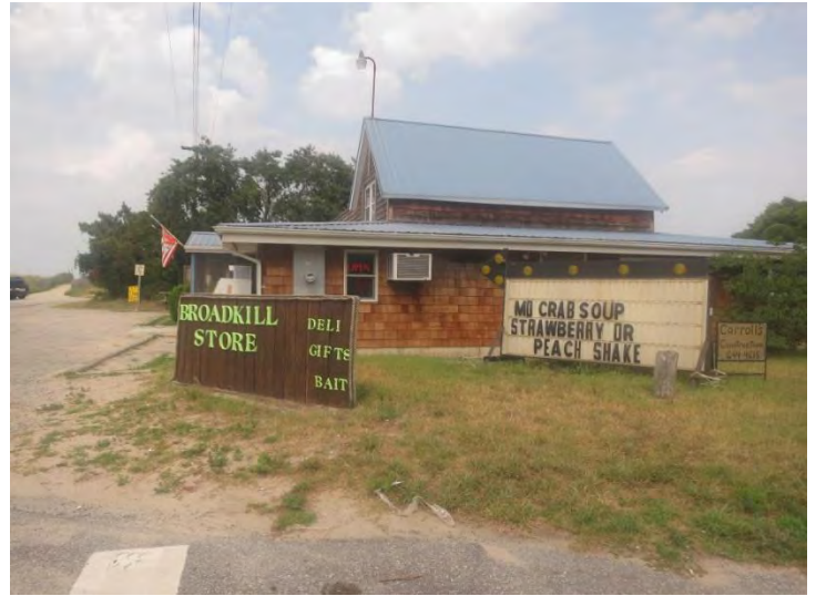
The only commercial building in Broadkill Beach sells deli items, beach supplies, and bait and tackle
