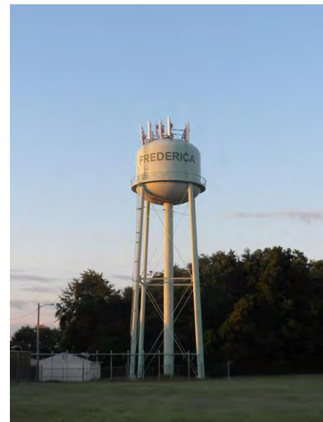
Town of Frederica Water Tower (Image Credit: Town of Frederica)
