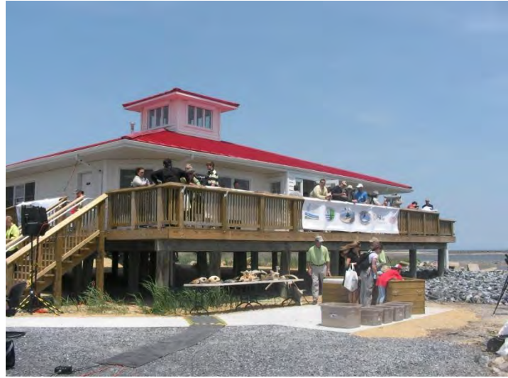
DNREC’s DuPont Nature Center at the Mispillion Harbor
