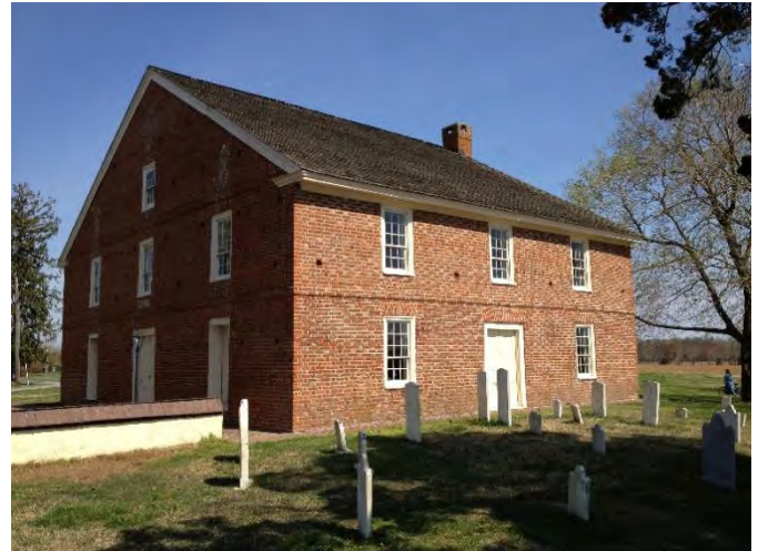
Barratt’s Chapel and part of its cemetery. (Photo Credit: Center for Historic Architecture and Design)
