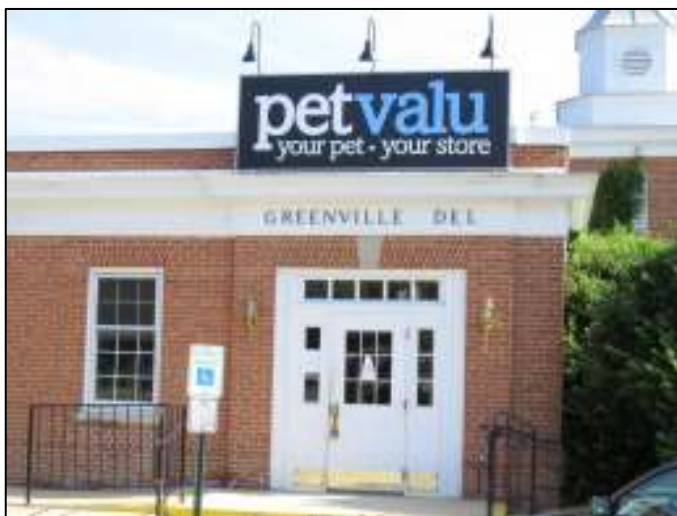
This Pet Valu sign violates the UDC and is not in the character of the Byway or the community. Source: KPA
