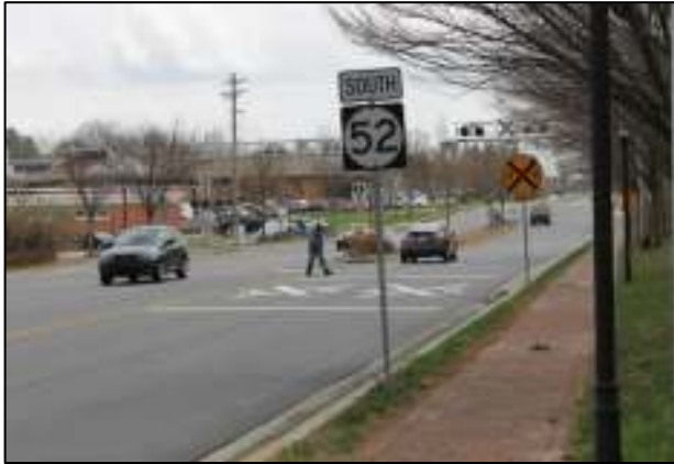
The railroad grade crossing of Kennett Pike in Greenville. Note the overhead lights and cross bucks protecting the crossing.
