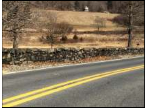
Stone walls along Route 100 on the Winterthur property.
