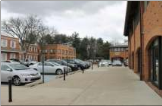
Greenville Center is a multi-building center. In this picture, there are office buildings across the parking lot from the retail building.
