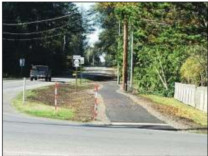
A context sensitive pathway is not at all like a sidewalk. As shown in the illustration, the asphalt pathway is aligned to avoid landscaping and is positioned to permit roadway drainage.
