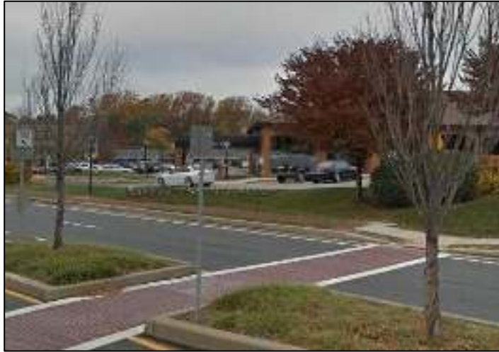
The brick crosswalk is a series of thermos-plastic tiles designed to look like brick and match the sidewalks. Used at each crosswalk in the commercial center of Greenville, the crosswalks connect both sides of Kennett Pike and are consistent with much of the building materials used in the center.
