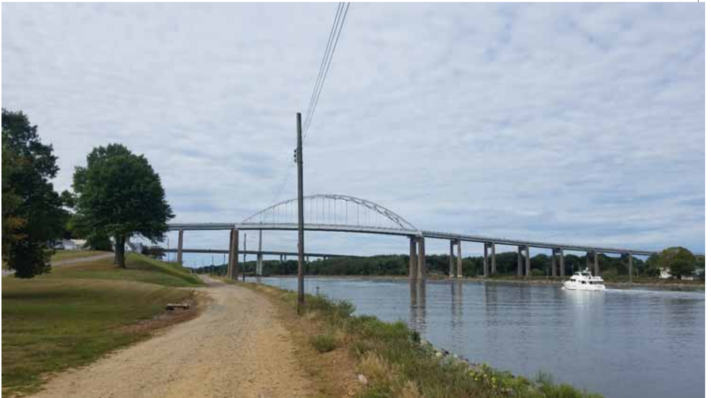
Figure 1: South St. Georges looking west towards the St. Georges and Roth Bridges.
