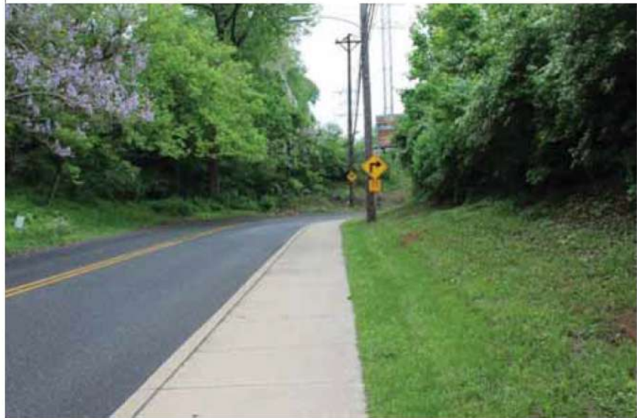
Figure 9: Existing sidewalk on the south side of West 18 th Street, looking east toward the curve in the road that travels under the railroad bridge. Extending the sidewalk into the grassy right of way to become a multi-use trail would likely require retaining walls and utility pole relocation.
