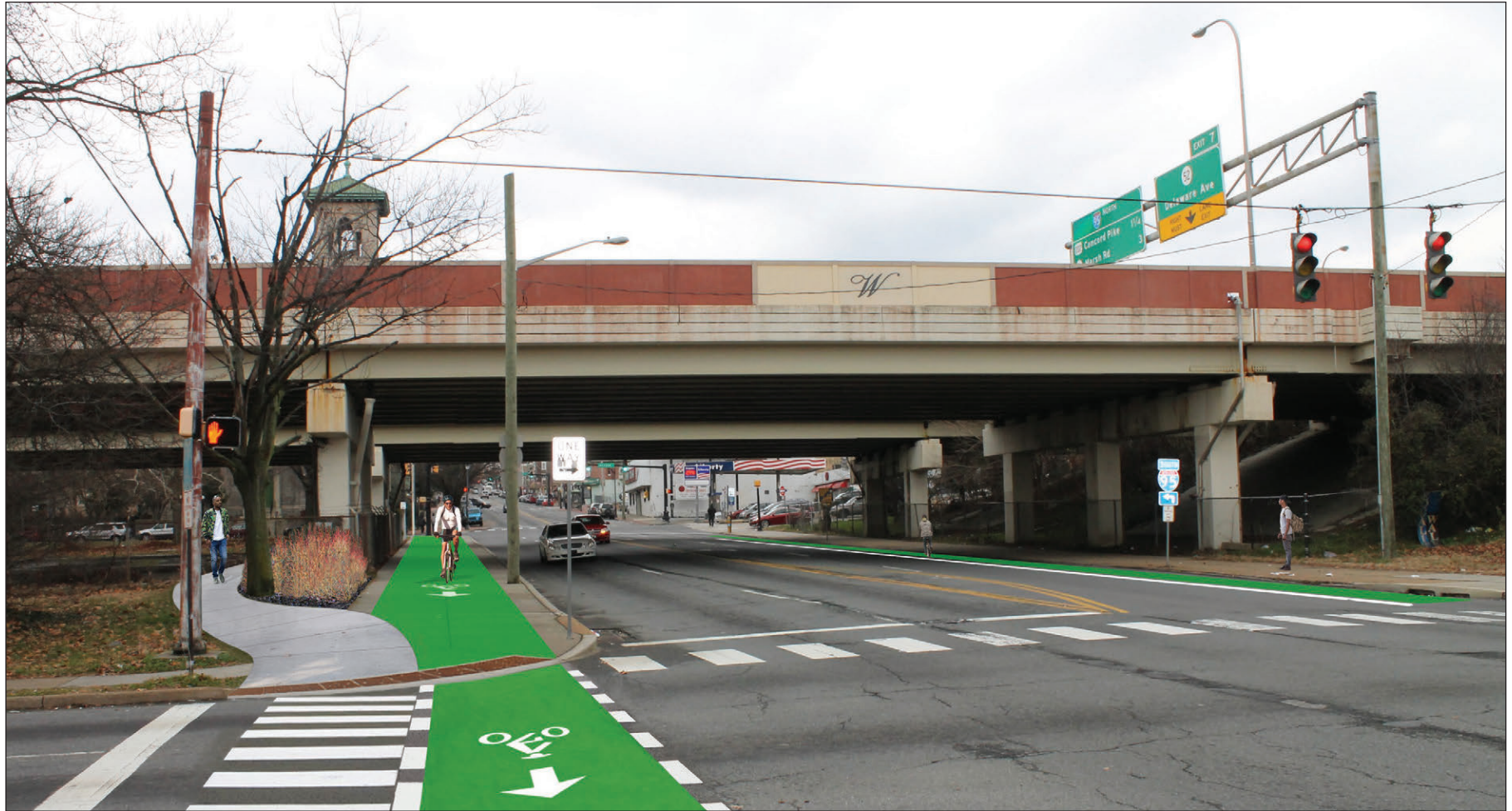
FIGURE 6: PORTION OF 4TH STREET CORRIDOR CONCEPT BIKE LANES AND SEPARATED PATHWAY ALONG 4TH STREET
