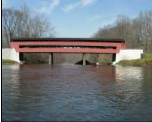
Smith Bridge located on Smith Bridge Road
