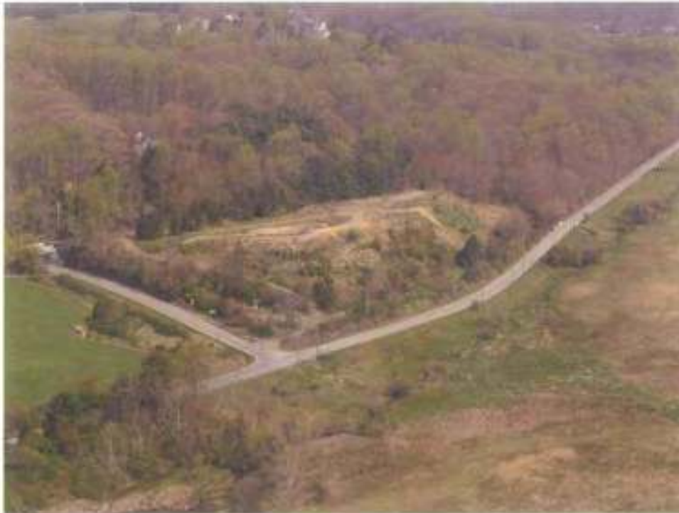
Plate 107. Rubble mound from the air
