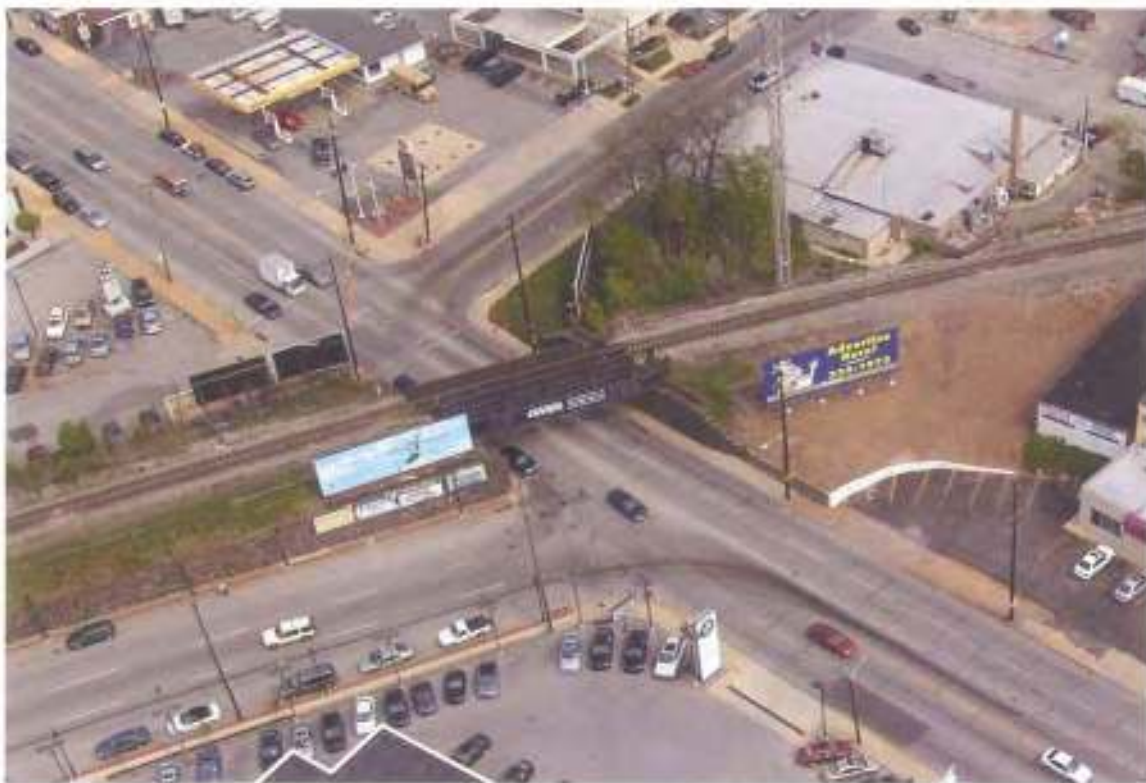
Plate 028 CSX railroad overpass at Pennsylvania Avenue
