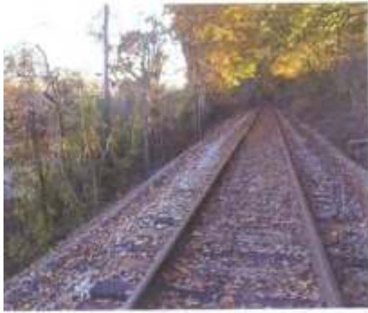
Plate 102 Wilmington and Northern railroad and its right-of-way
