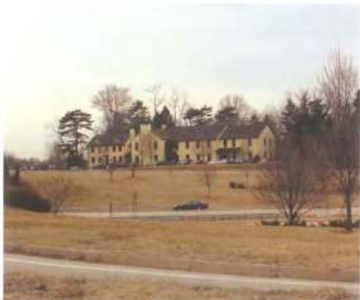
Plate 049 Interchange at Route 141 and Kennett Pike
