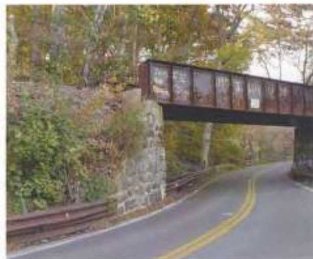
Plate 098 Wilmington and Northern railroad overpass
