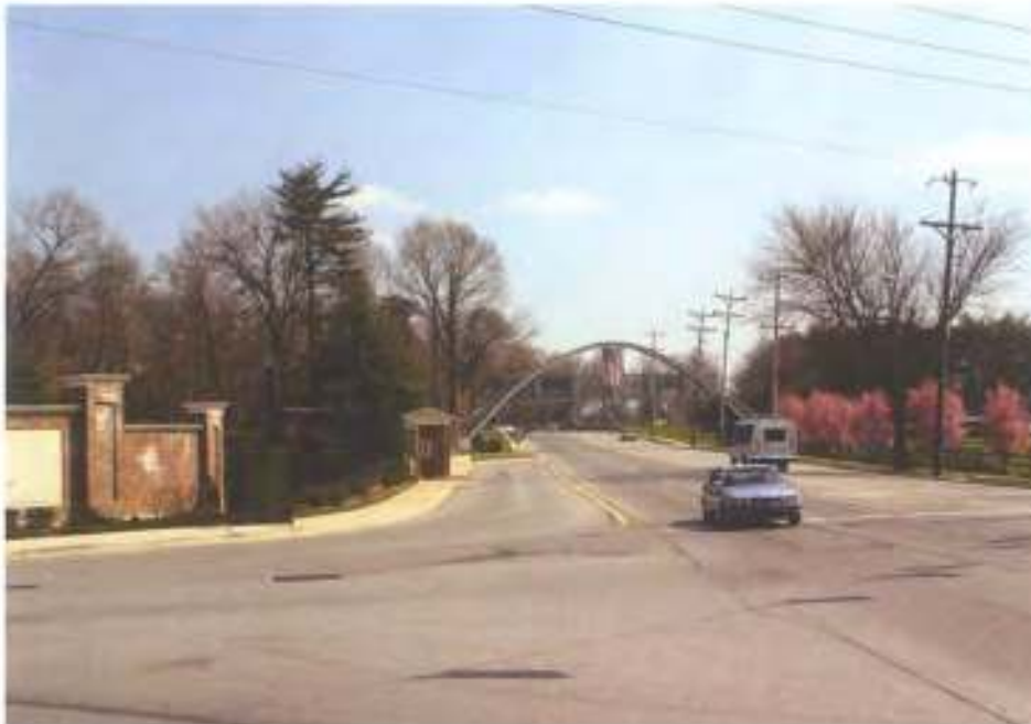
Plate 034 Tower Hill pedestrian overpass on Pennsylvania Avenue
