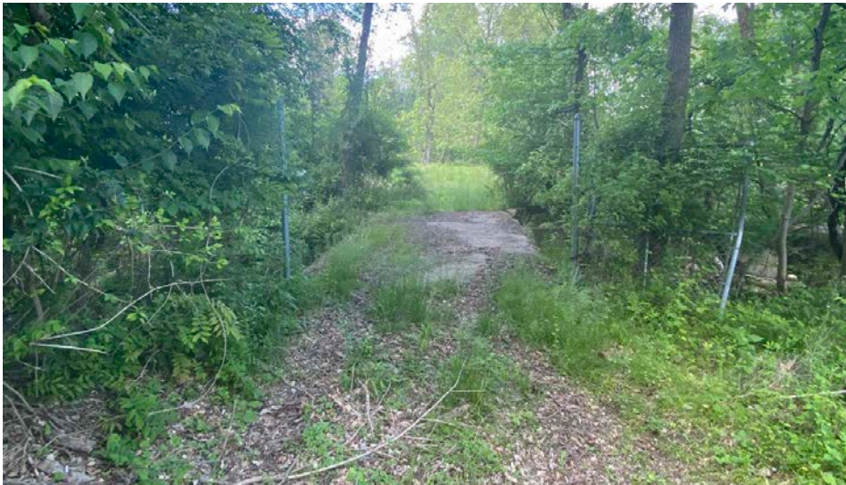
Photo 4: View of existing bridge crossing over Hyde Run
