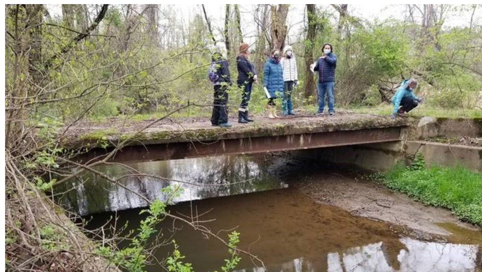
Photo 19: View facing upstream toward the existing bridge
