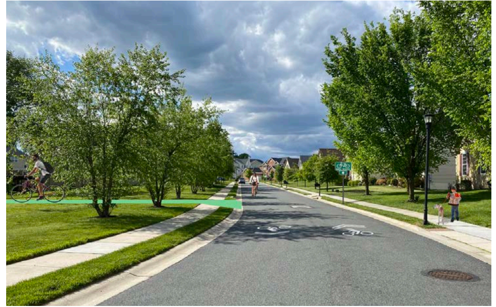
Figure 28: Photo sketch of signed shared lane markings on Oracle Road with existing sidewalks in Greenville Overlook development for alignments B2 and C2
