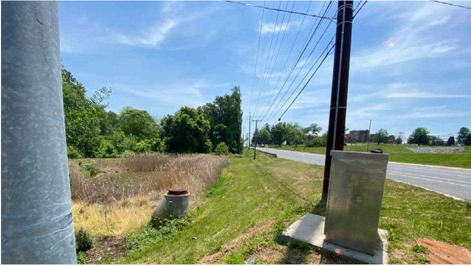
Photo 11: View of utilities at the southeast corner of Newport Gap Pike and Millcreek intersection with slope challenges along stormwater management facility
