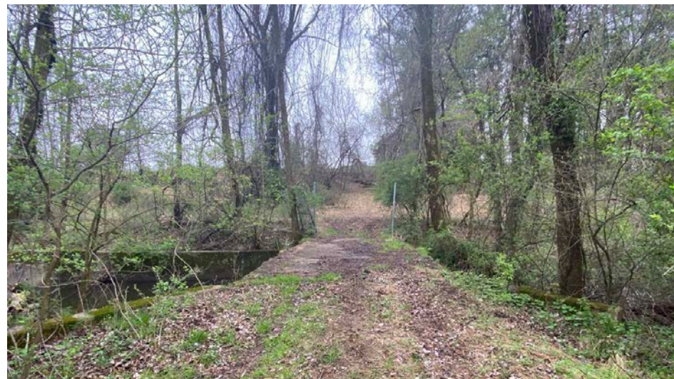
Photo 18: View from the existing driveway on the west side of the existing bridge
