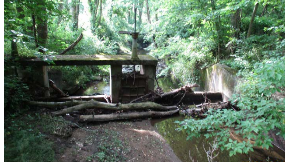
Photo 22: View downstream of retaining walls and weir structure
