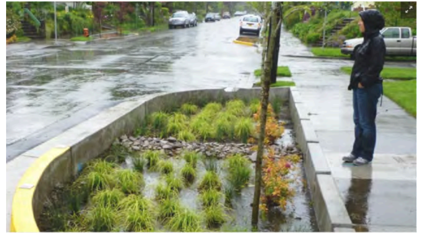
Bioswales have many benefits, including a reduction in strain on a city's municipal sewer system. Less water in sewers generally leads to cleaner rivers and waterways. Click through the gallery for more about Portland's bioswales.
