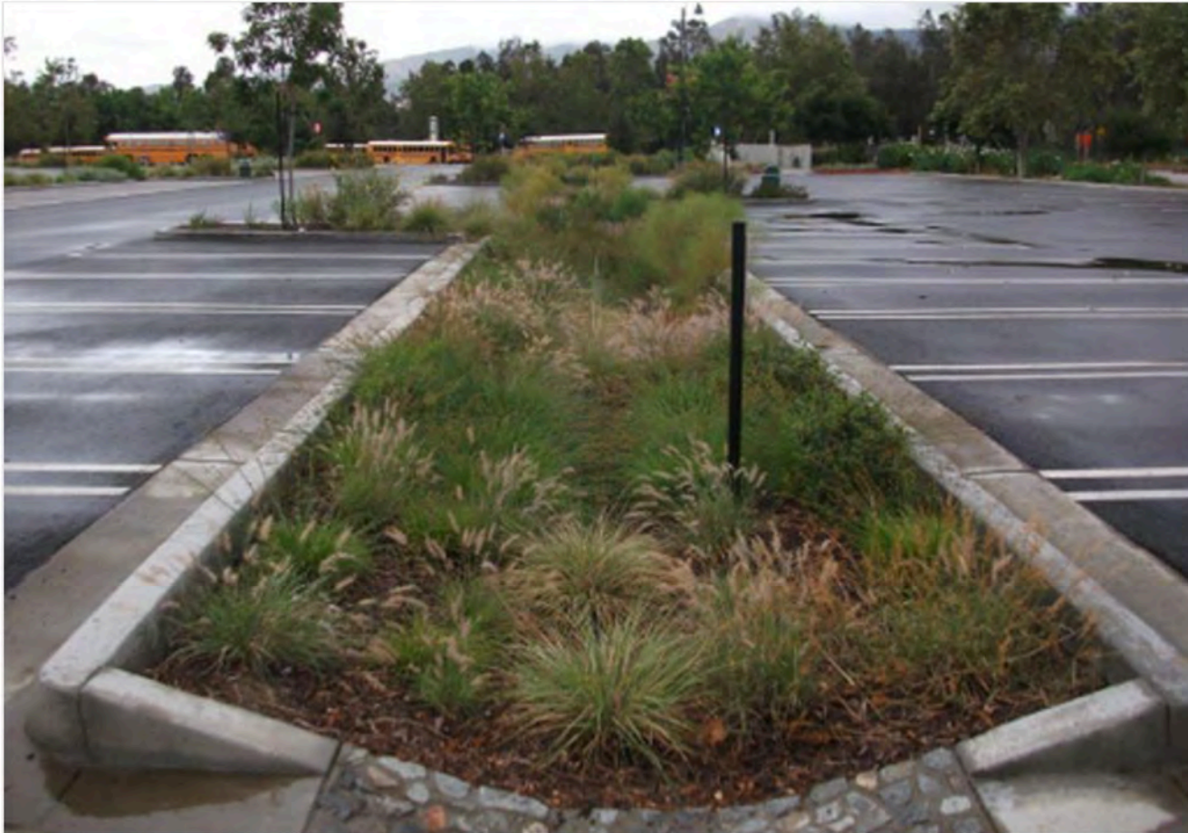
This is a bioswale at the L.A. Zoo. By centering it, run off is collected from both sections of the parking lot.
