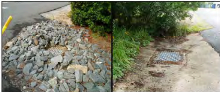
Figure 9. Inlets surrounded by rip-rap and concrete in N4 (South Bethany) that can be modified to remove the impervious cover and include grass/native vegetation pretreatment.
