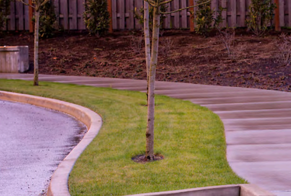
Bioswales have many benefits, including a reduction in strain on a city's municipal sewer system. Less water in sewers generally leads to cleaner rivers and waterways. Click through the gallery for more about Portland's bioswales.
