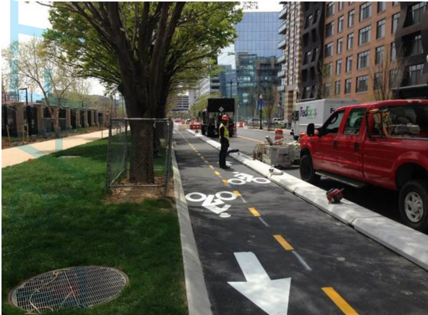
Raised Bike Lane
