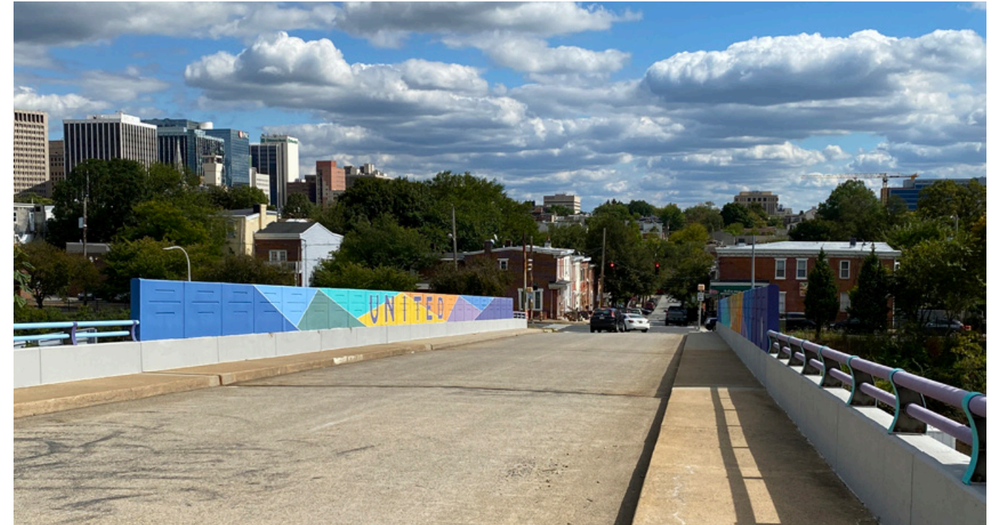
The W. 7th Street Bridge looking East at Adams
