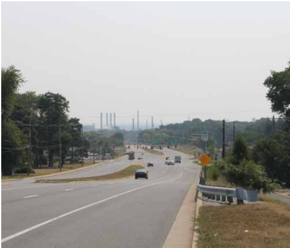
View toward the Delaware River from Naamans Road west of I-95
