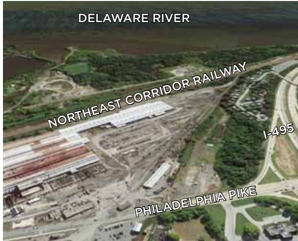
Former conditions near proposed train station site (facing south)
