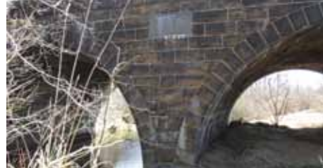
9. Bridge on mill site
