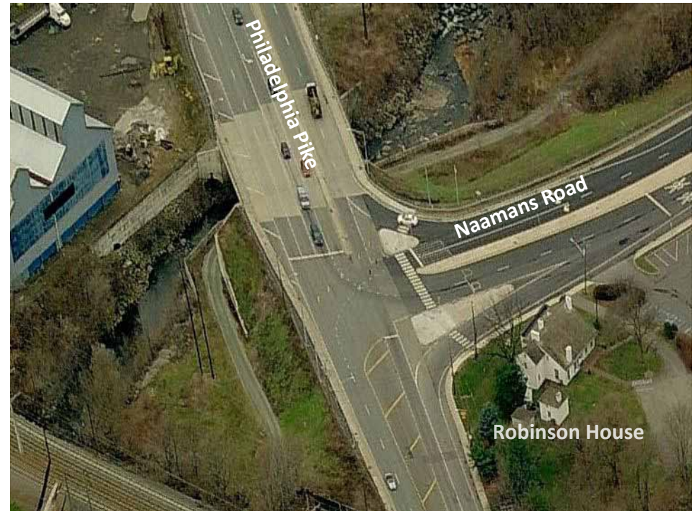
Existing conditions at Philadelphia Pike and Naamans Road
