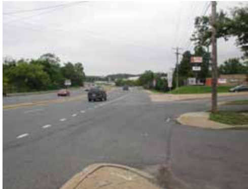
Though there is a sidewalk on the north side of Naamans Road, it is often disconnected.
