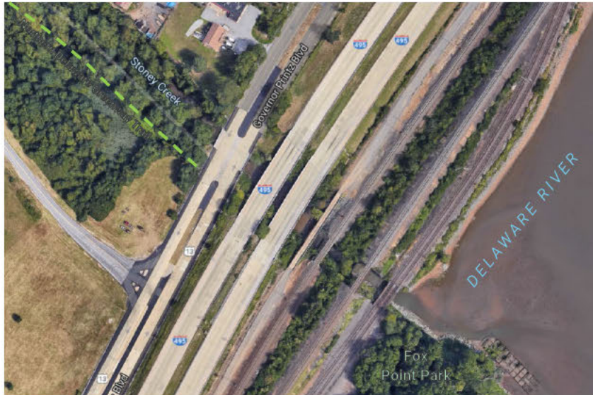
Figure 27. Aerial photograph showing infrastructure in the vicinity of Stoney Creek. Source: Google Maps.
