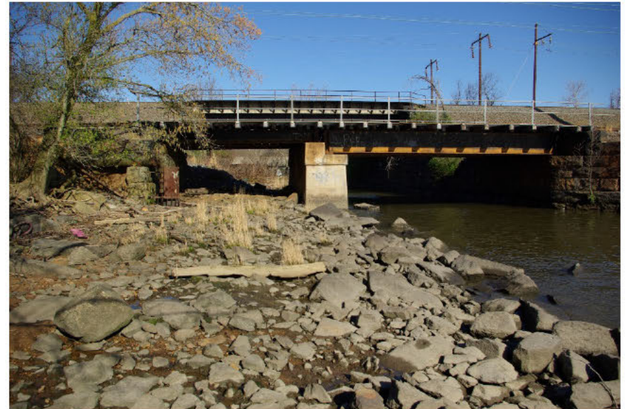
Figure 28. Norfolk Southern Bridge looking northwest up Stoney Creek
