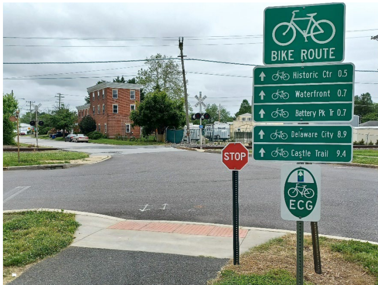
Figure 16. Standard MUTCD compliant wayfinding signage in New Castle, Delaware. (Source: Delaware Greenways)
