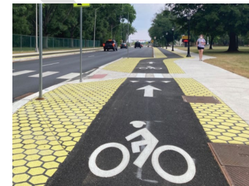
Example of Sidewalk-level Bike Lane (Newark, DE)
